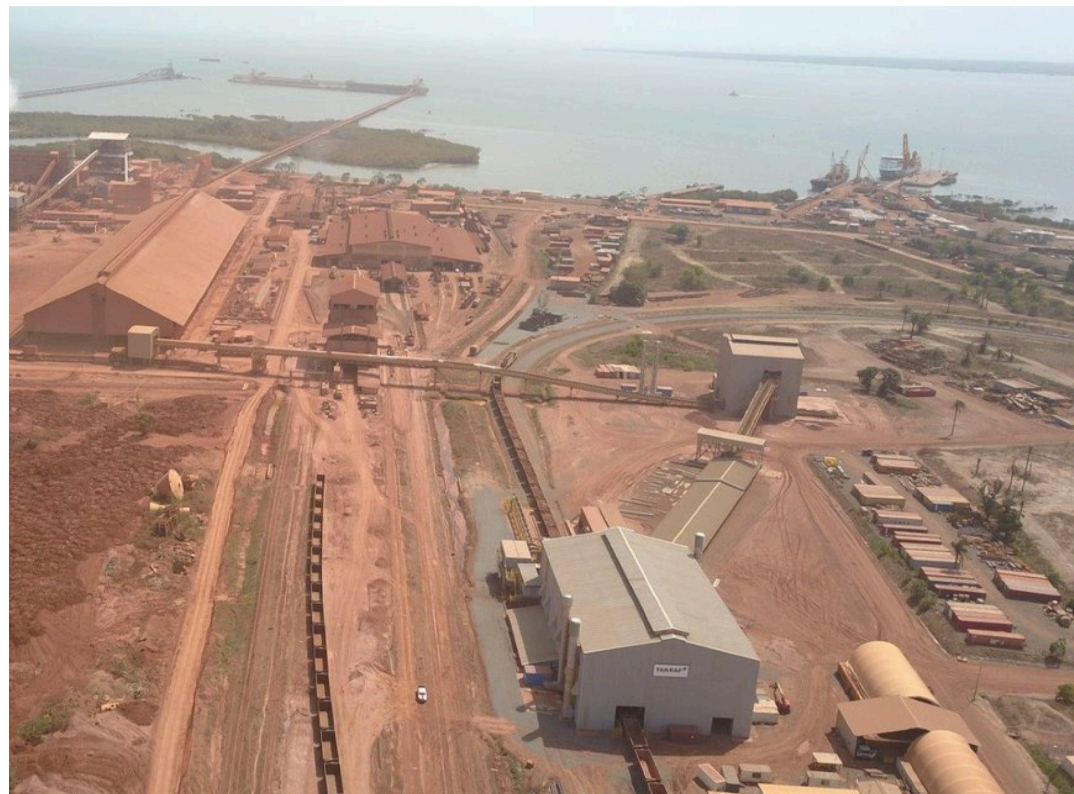
An aerial view of the overall plant in Guinea with the wagon unloading station building from Phase 1 in the foreground.
