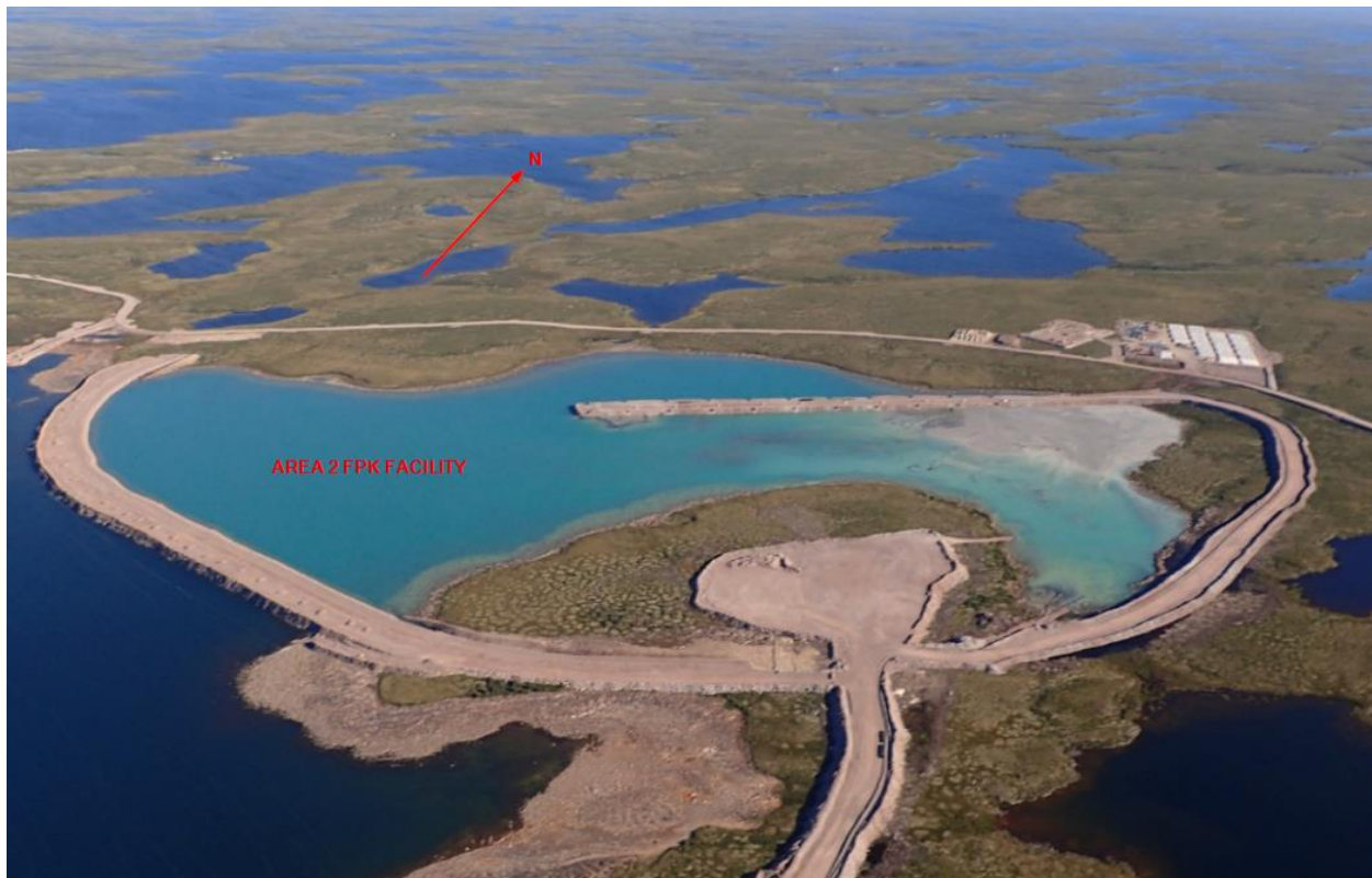
Figure 17-4: Area 2 Fine Processed Kimberlite Facility
